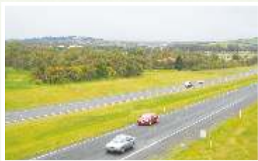
Calder Freeway with Sunbury in background
